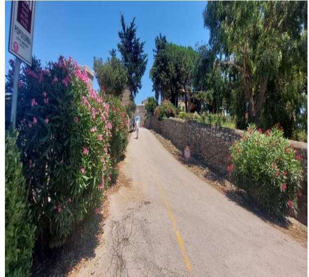
6 Asphalt entrance ramp, from the car park.
