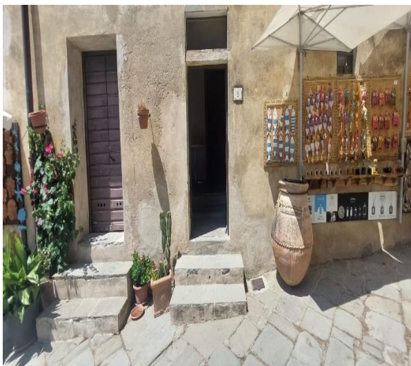
57 Toilets not accessible
