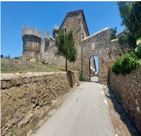
7 final section ramp
